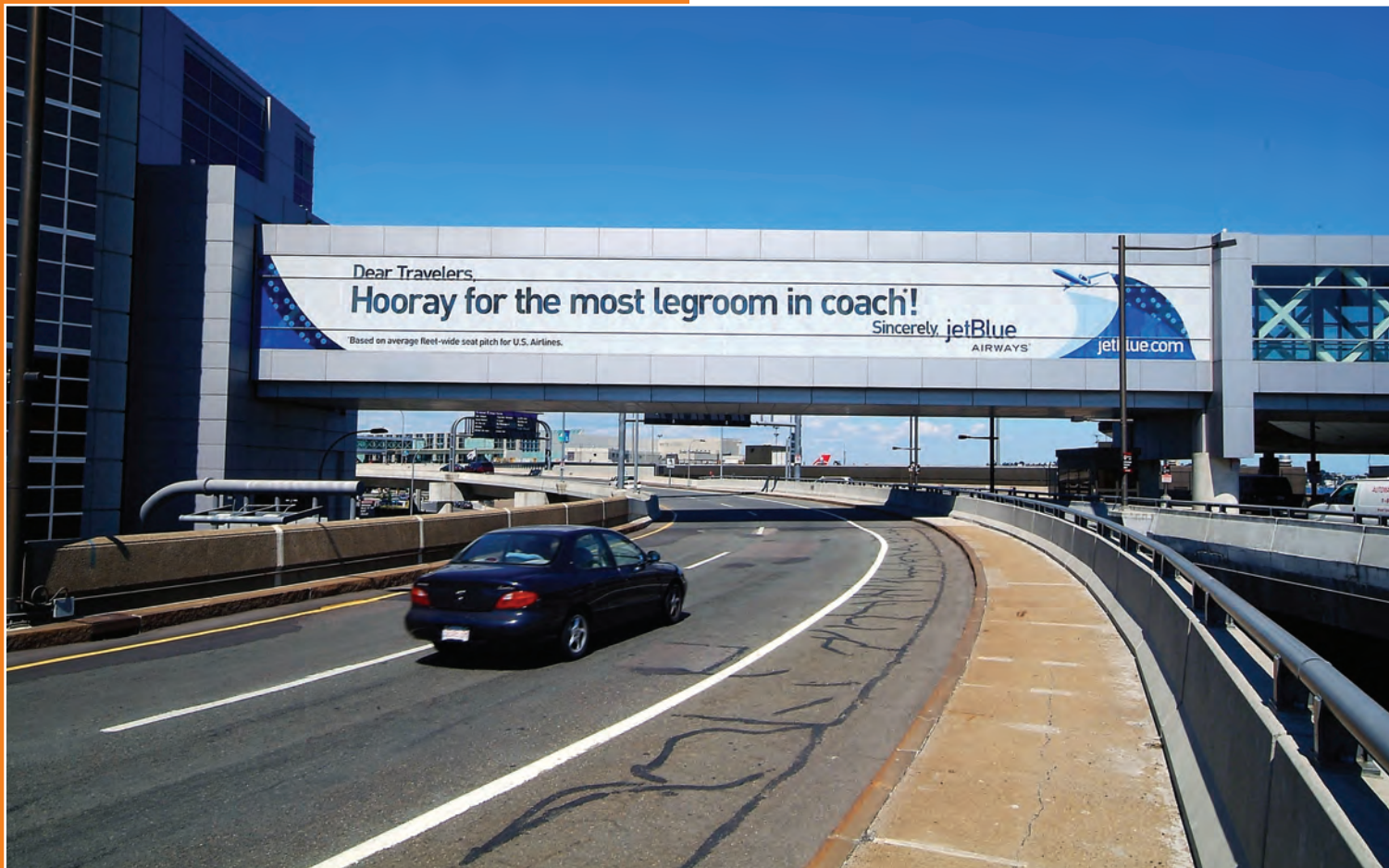
Pedestrian Bridge Cling - Boston Logan International Airport
